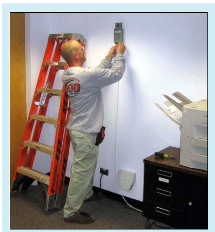
Bryan Anderson, a Network Technician with NETS, installs and configures one of the Cisco wireless access points to upgrade the Local Area Wireless (LAN) system for all UCAR campuses. This upgrade gives NCAR/UCAR staff broader, faster, and more reliable wireless connectivity to local networks and the internet.
